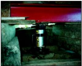
Choose light weight aluminum cylinders when easy carrying and positioning are important. Here Simplex RAS-Series aluminum cylinders were specified to overcome a difficult setup in tight quarters while leveling a large structural foundation. See page 15.
