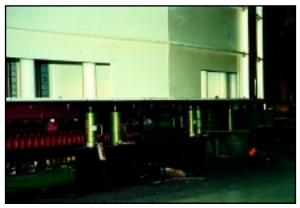
RLN Series lock nut cylinders cut installation time on this power generator by 25%. "The locknut held the load without the extra chore of cribbing." The job was completed even quicker with the use of Simplex SUC-O-MATIC<sup>™</sup> power pumps.
