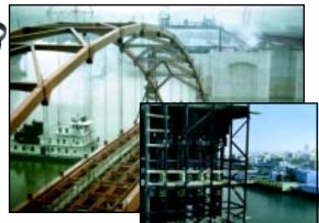
Engineers from around the world watched as Simplex center hole cylinders raised a 6,000 ton bridge section more than 170 ft. over the Willamette River in Portland, OR. The span was constructed up river and barged into position. Using pull rods and couplings, Simplex RCD200 Series cylinders completed the lift in 40 hours.
