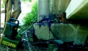
Construction Sites, Ship Yards, Railroads and Other Field Applications require portable pumps that start and run on less than ideal power conditions. The 70 Series pump incorporates a powerful 1.5 HP Permanent Magnet motor that will start under full load and run reliably on long extension cords & reduced voltage. This is the new standard for construction applications.
