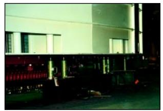
Choose locknut cylinders when the load must be lifted and held in place for a period of time. In this application Simplex RLN-Series cylinders cut installation time on this power generator by 25%. "The locknut held the load without installing cribbing." See pages 26 - 27.
