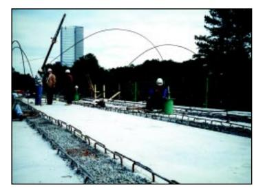
These construction crews use Simplex Hard-Kor<sup>TM</sup> hollow cylinders to pre-tension steel rods in cast concrete forms. "The Hard-Kor<sup>TM</sup> cylinders, with their leak-proof base and extra power, made a tough job easy."
