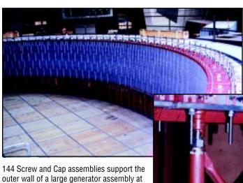
144 Screw and Cap assemblies support the outer wall of a large generator assembly at the Grand Coulee Dam. The assemblies also are used to exert pressure, stabilizing the generator laminations.
