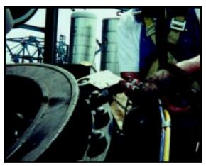
When this power plant needed flange maintenance, engineers called on Simplex for solutions. Changing out flange seals requires precision torquing and minimal down time. Simplex power units and low clearance wrenches filled the plant's needs, saving significant cost and down time.
